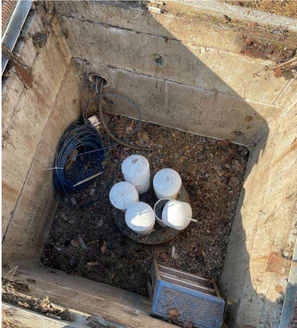
Image of a Transducer Well access vault in the Chino Basin
